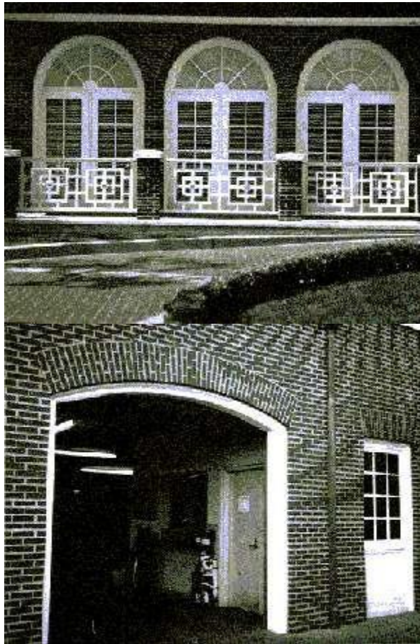
Structural Brick Arches FIG. 1
