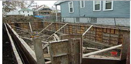
Steel and plywood formwork
