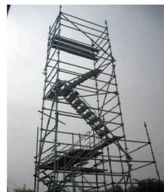
Braces to standards
