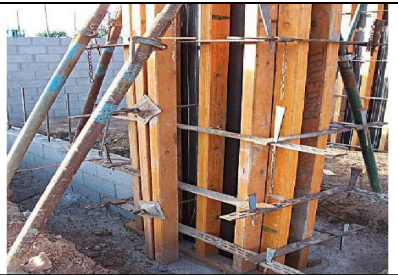
Steel and plywood formwork
